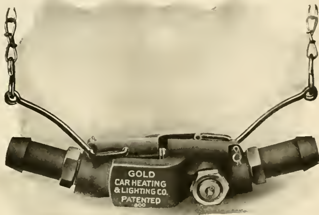
AUTOMATIC LOCK AND HOSE SUPPORT
